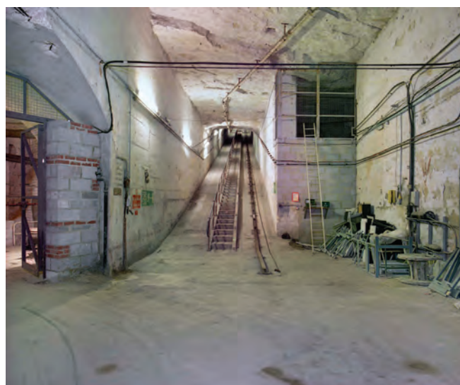
Tunnel Quarry at Corsham, Spring Quarry is at the top of the slope. Photo Nick Catford
